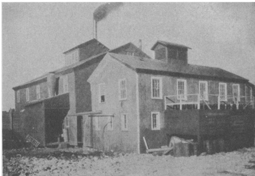
Oil refinery plant.
